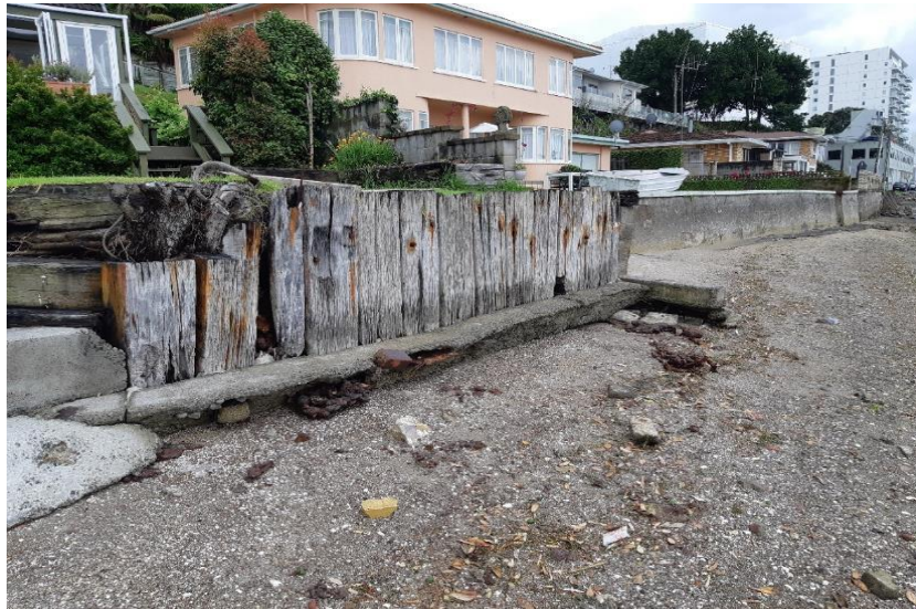
Existing seawall to be replaced.
