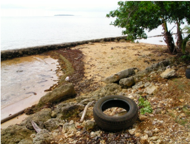
Figure 2 A tombolo formed in the lee of a failed seawall at eastern Manuka.
