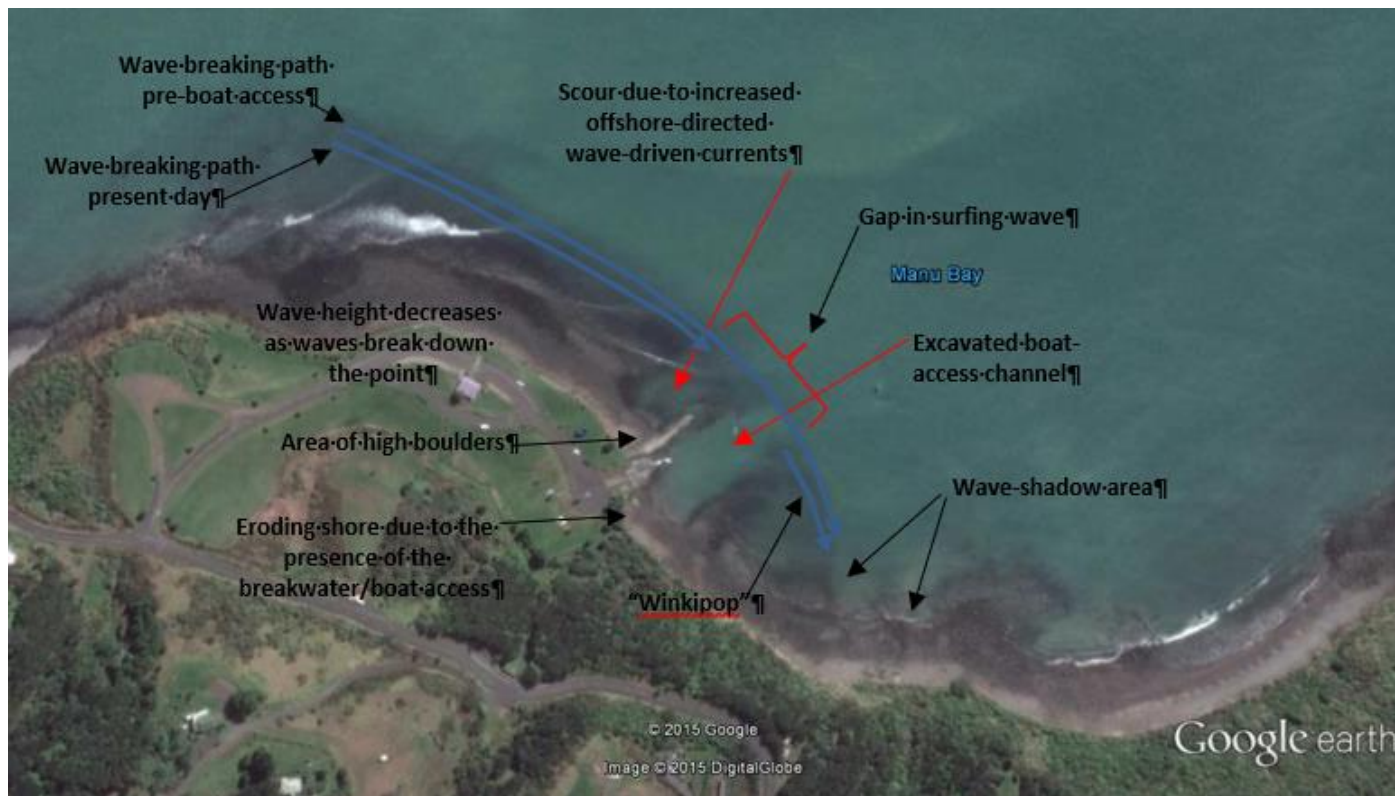
Image of Manu Bay, Raglan showing the decreased surf zone due to the excavation of the boat access ramp and scour of the north-western side of the breakwater.
